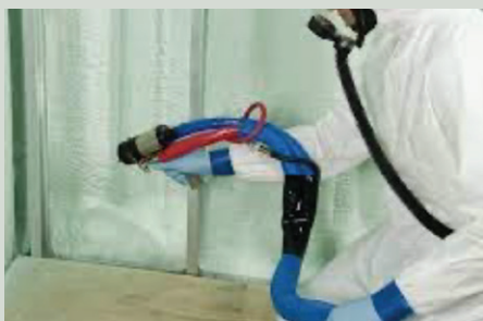
Figure 2: Application of SPF between Timber studs (photo courtesy of Huntsman Polyurethanes).
