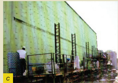
Figure 3: a) The “Clever Wall” utilising SPF as insulation, water, air and vapour barrier, from The Condensation in Buildings Handbook provided by the Australian Building Codes Board under the CC BY 4.0 licence. b-c) application of SPF.
